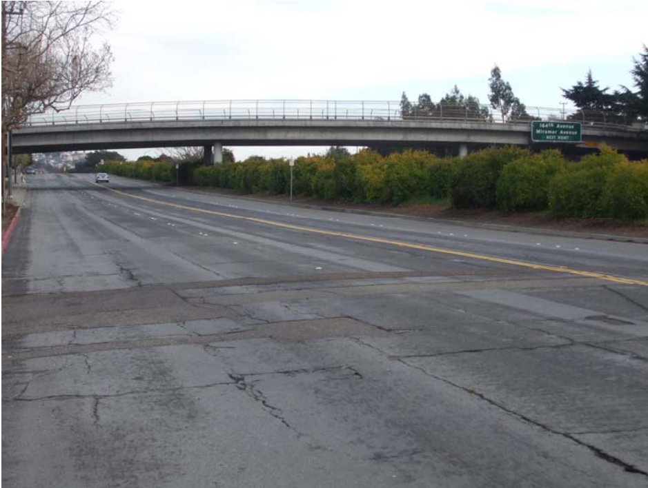
Foothill Blvd/159 th Ave. Overpass (Southbound view)
