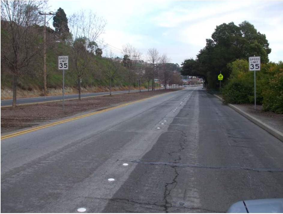
Foothill Blvd near Carolyn St. (Southbound view)
