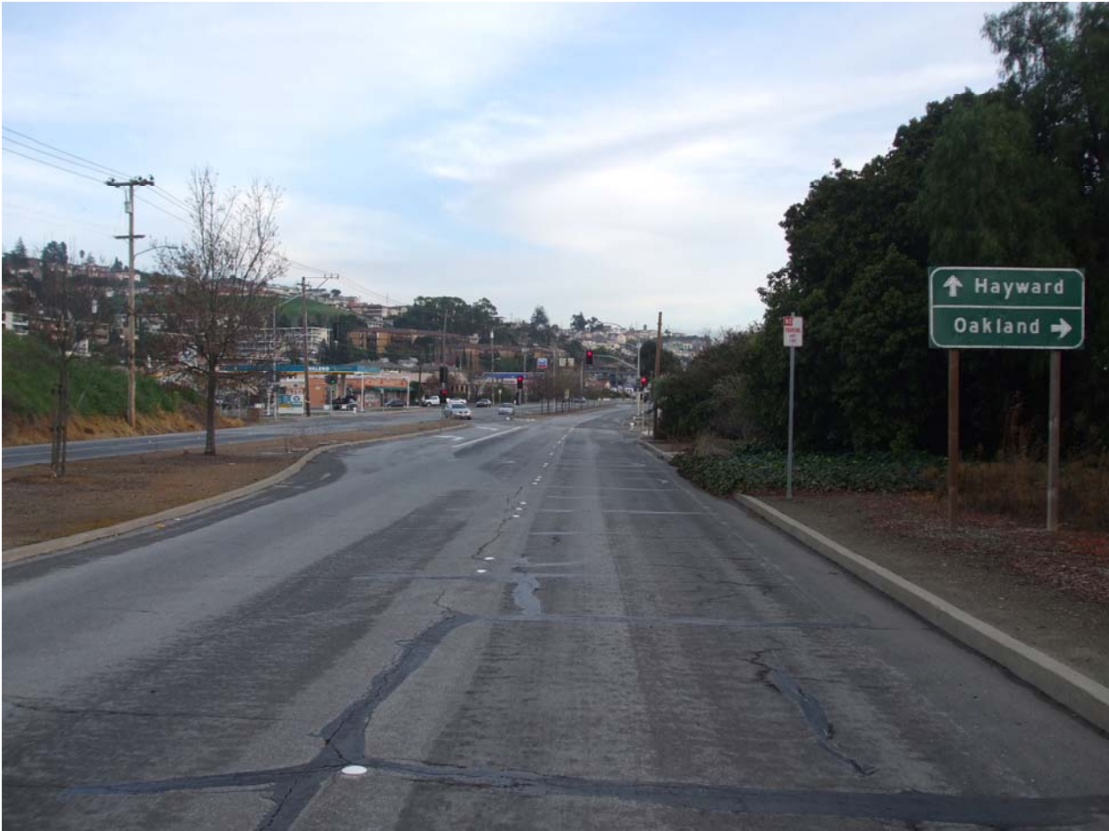
Foothill Blvd / Carolyn St. (Southbound view)
