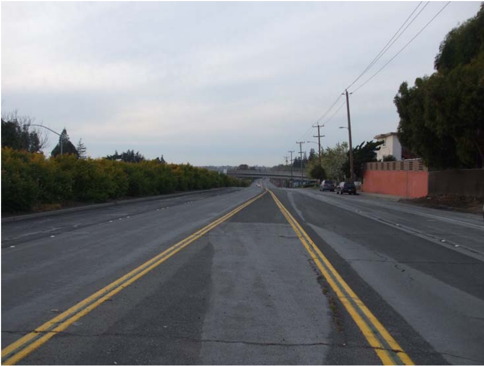
Foothill Blvd near Manchester Road (Northbound view)
